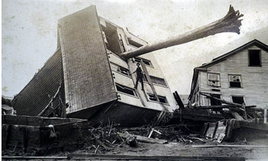
The Schultz home was found one-half mile from its foundation with a tree sticking out of it. All six members of the Schultz family survived.
